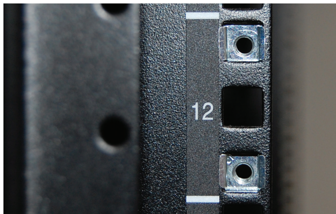
FIGURE 2-1. INSTALL THE CAGE NUTS
